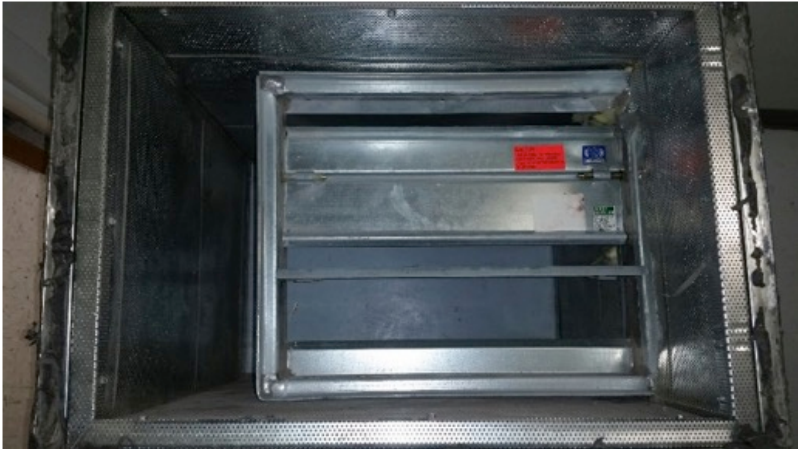
Damper Smaller Than the Duct
