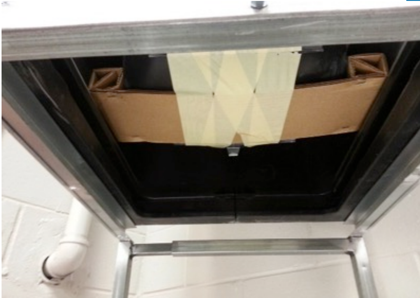
Packing Material Left in Unit
