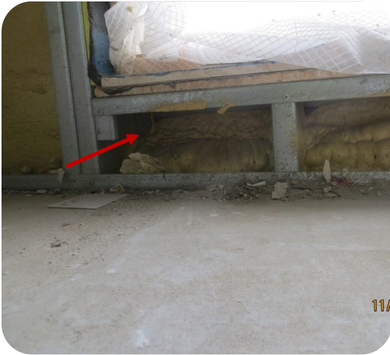
Insufficient spray foam
