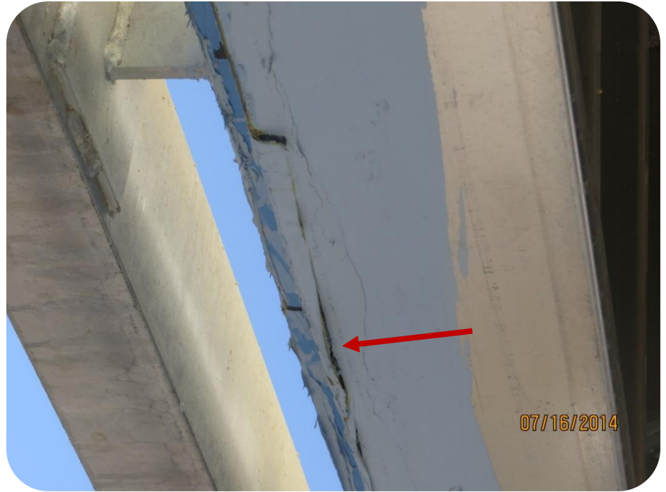
Unadhered flashing
