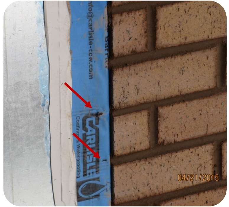
Holes in flashing
