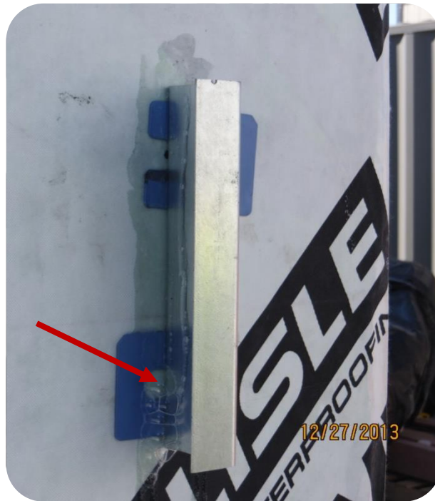
Z-girt fasteners
