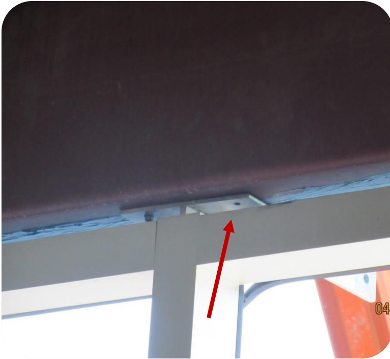
Curtain wall fasteners
